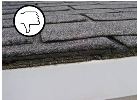
Example of Multiple layers Comp Shingle
